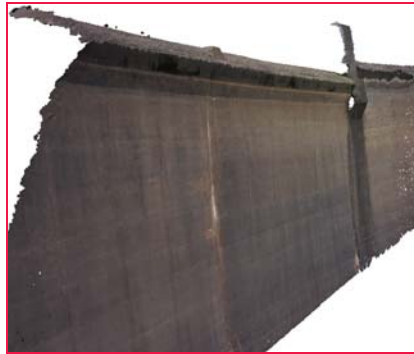
Figure 26: Point cloud of a section of the spillway
