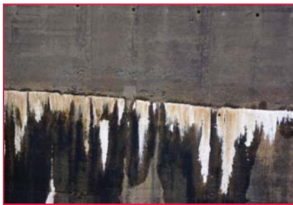
Figure 24: Horizontal photograph of the downstream wall of Bouça dam
