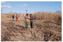
Figure 5: Drilling site stakeout: set out the site to the actual position, the two workers at the back mark the drilling site position with a wooden pile and red cloth.
