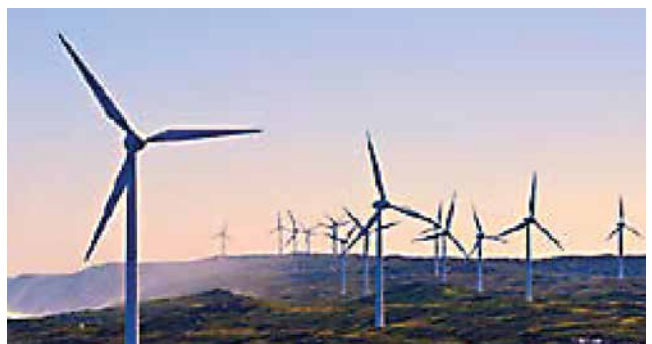
Figure 7: A typical wind farm with wind turbines (courtesy Reglobal analysis as in nature journal of science)
