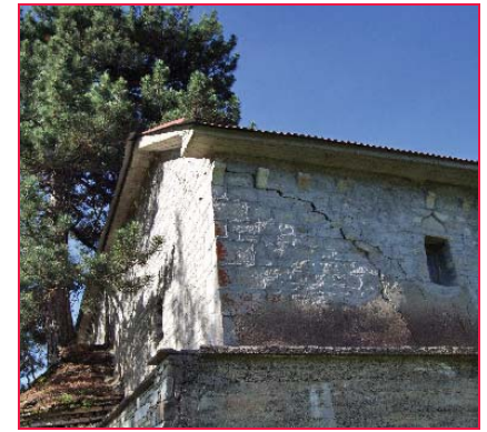
Picture 4: Damage caused by structural deformation
