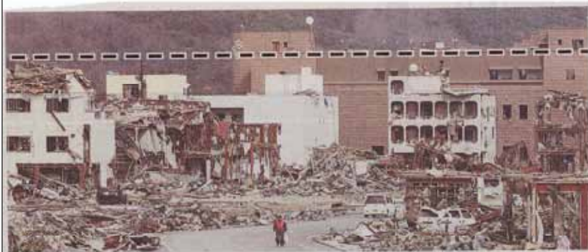
Fig.5 Water Level of Tsunami (15m) in Onagawa Town Up to the Roof of the Fifth Floor Building
