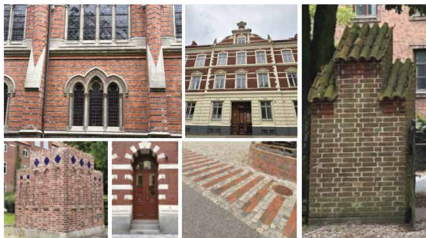
Fig. 2. Examples of brickwork and organic architectural structures from the past.
