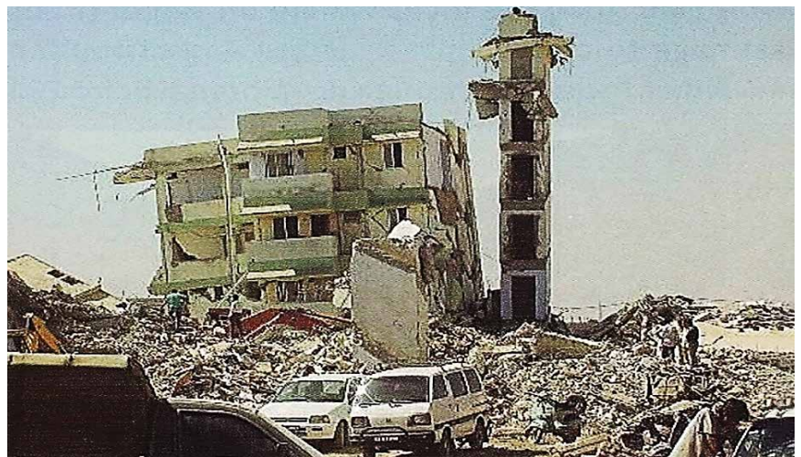
Fig. 1: The Gujarat earthquake on 26 January 2001 left over 20,000 people dead and more than 1,65,000 injured.
