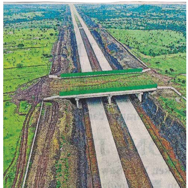
Fig. 28: Highway/Railway Lines may be provided with an Overpass for Safe Crossing of Villagers, Animals, etc
