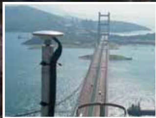
Continuous Monitoring of Bridge Movements
