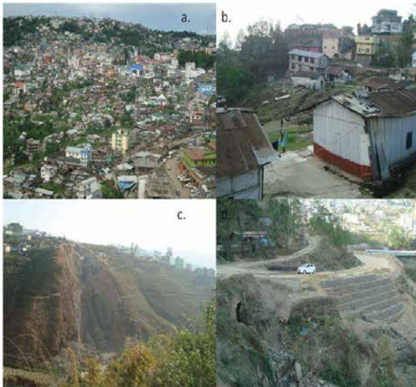
Figure 5: a). Portion of the study area- note the closely constructed heavy concrete construction on unstable slope. b). Affected buildings in Ward no.1 of the study area. c). Landslide with an approximate length of 150 m in Ward no. 6. d). Landslide at Asian Highway (AH) 1 in Ward no. 18.
