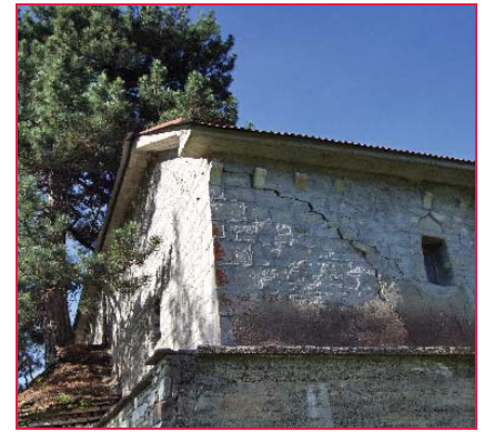
Picture 4: Damage caused by structural deformation
